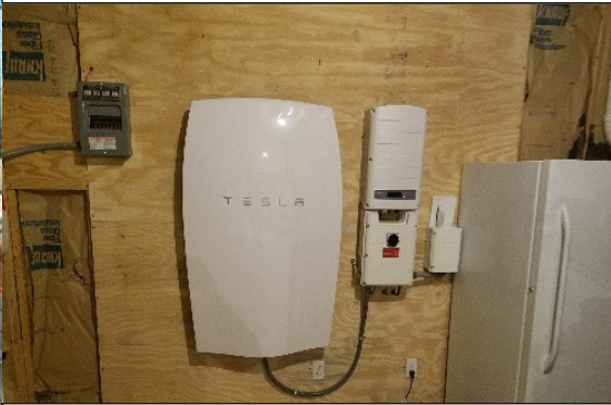
Tesla Powerwall unit installed by Peck Electric in S. Burlington.
