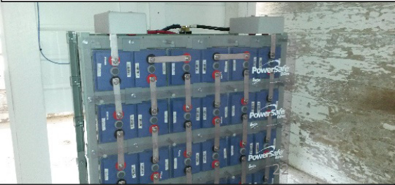
PowerGuru 32 kWh battery in Pownal
