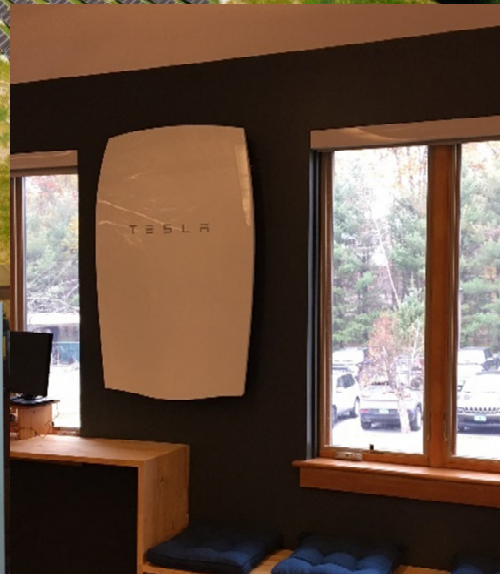
GMP Tesla Powerwall 5.5 kW install
