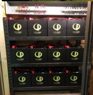
Simpliphi 82 kWh system at Emerald Lake
