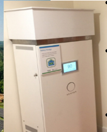
Vermont Sonnenbatteries (6 or 8 kWh) at McKnight Ln. project in Waltham
